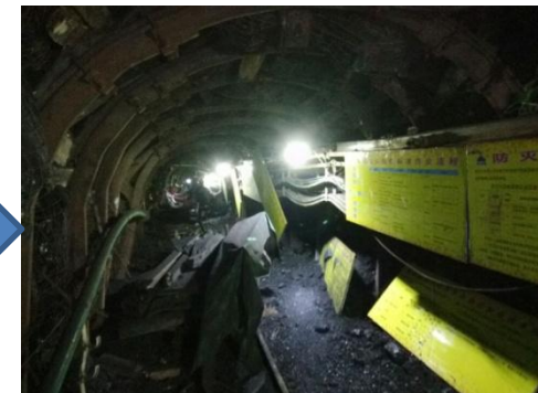
Plate falling off
