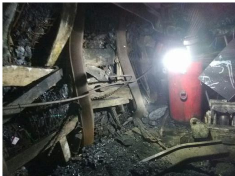
Bottom distortion of U-shaped steel
